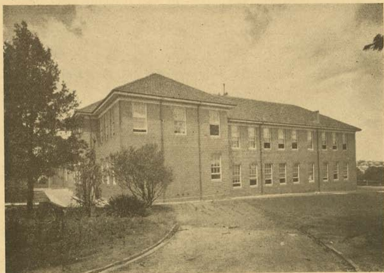
NORTHERLY VIEW OF SCHOOL.
