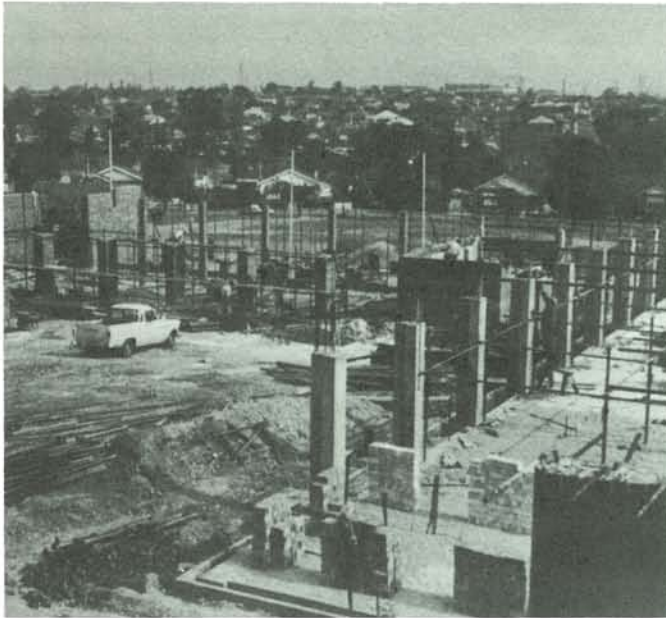
Progress on the new buildings.
