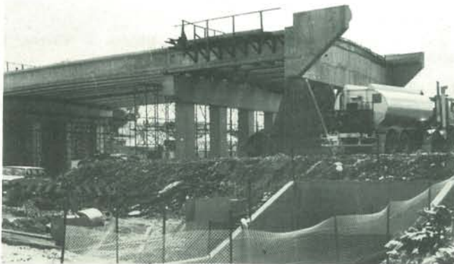
Construction of bridge over Underwood Road.
