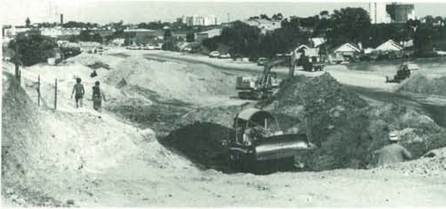
F4 — WESTERN FREEWAY
