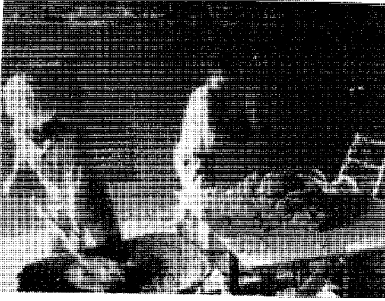
"Mud pies" - render being applied to brickwork.
