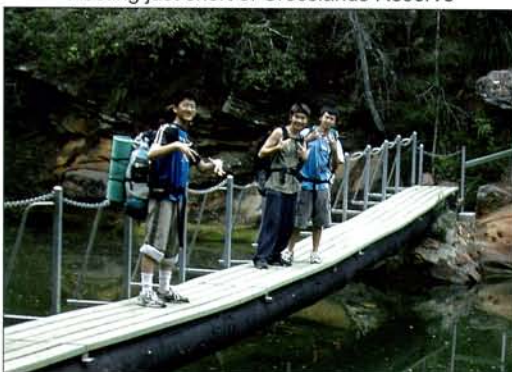
Calna Creek Bridge
