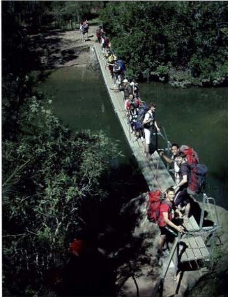
Calna Creek Bridge
