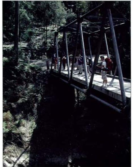
The Bailey Bridge over Berowra Creek
