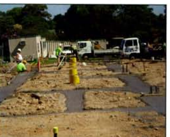
Concrete poured on footings.
