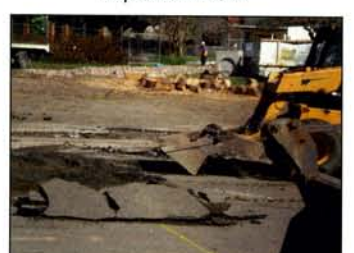
More concrete to pull up.
