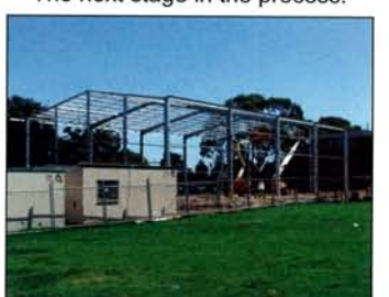
Work in progress October 2008
