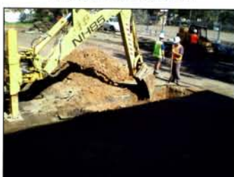
Digging the trenches.
