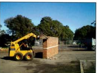
The wall has to go.
