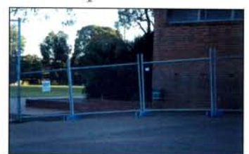
Safety fencing in place.
