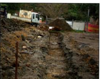
The trenches are prepared.
