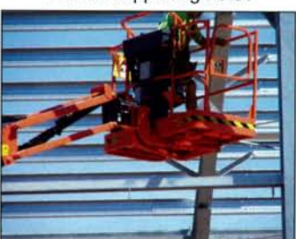
Crane works on frame.
