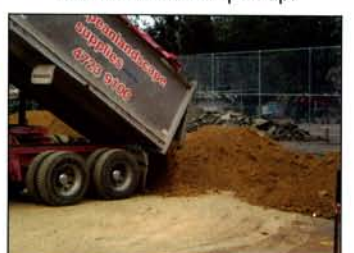
Trucks dump dirt.
