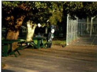
Workmen remove 'picnic' tables.
